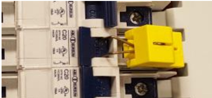
Fig. 3.3.3 – LOCKOUT Adapter Attached
