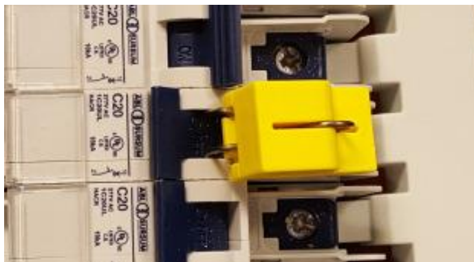
Fig. 3.3.4 – LOCKOUT Adapter in Place
