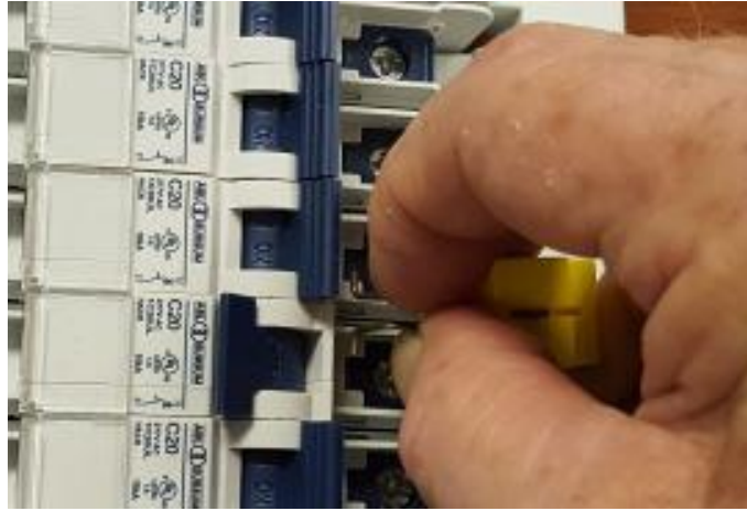
Fig. 3.3.2 – Applying LOCKOUT Adapter
