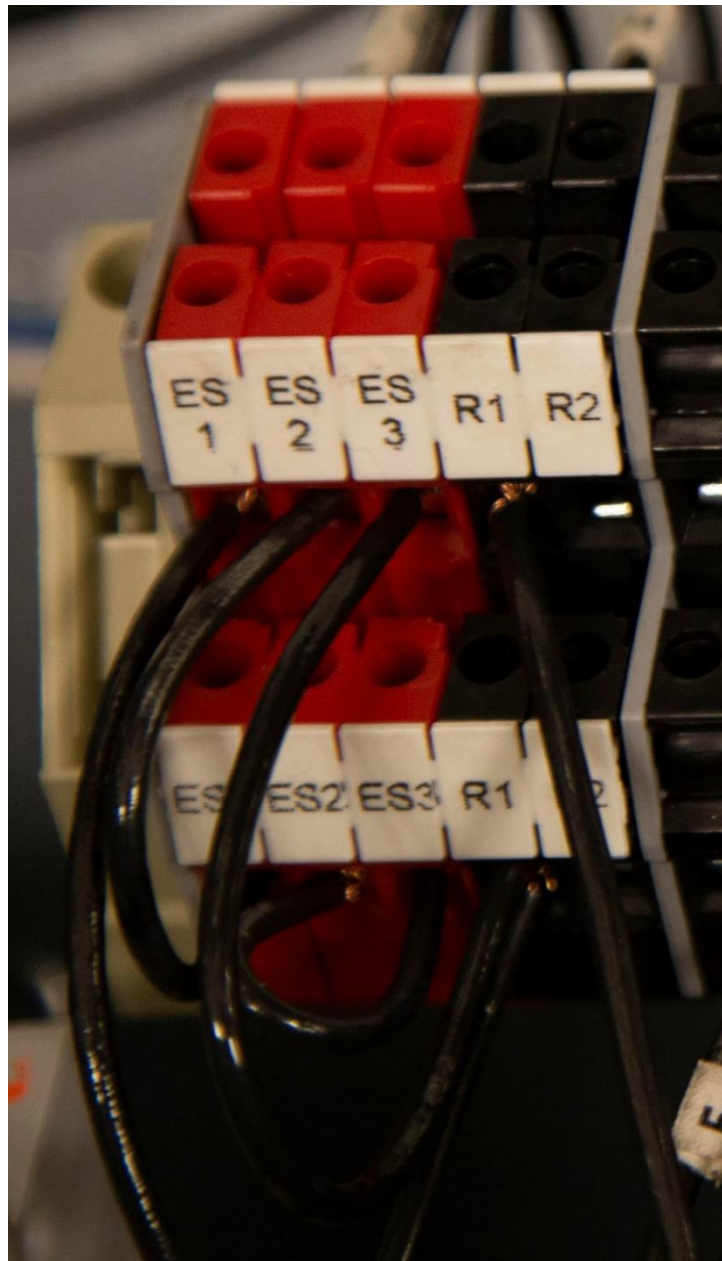
Fig. 1.2.2 – Wired FUELING SHUTDOWN and FUELING RESET Terminals
